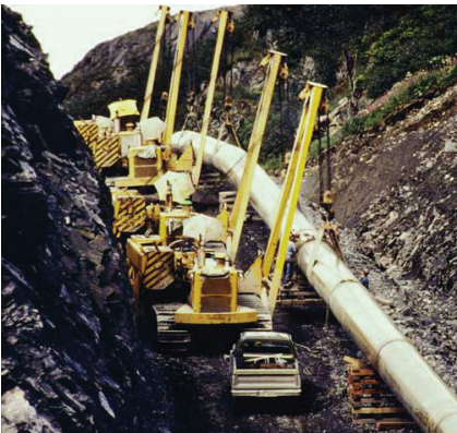
Trans-Alaska Pipeline construction through mountain pass, 1976. ALASKA STATE LIBRARY, HISTORICAL COLLECTIONS.
